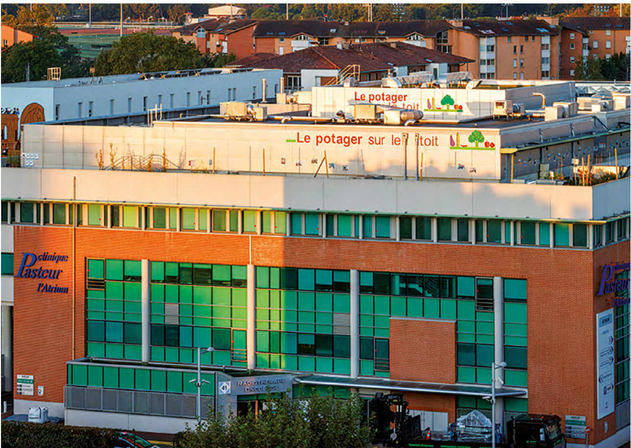
A view of the the Pasteur Clinic rooftop garden
