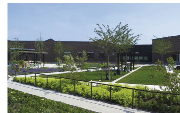
Trelleborg Passive House, Region Skåne
